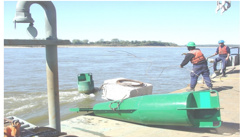
Crew members retrieving a floating ATON and preparing to deploy a new sinker and ATON. Photo provided by USCG.
