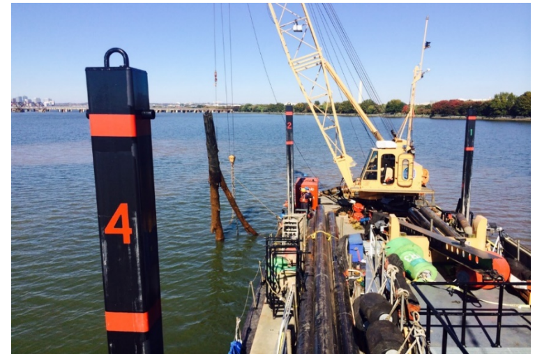
The crane of a WCC Construction Tender being used to remove a damaged fixed ATON. Photo provided by USCG.
