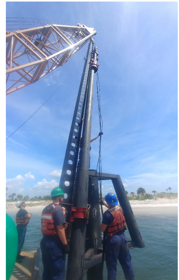
Crew members assist the attachment of the impact pile driver to a pile.
